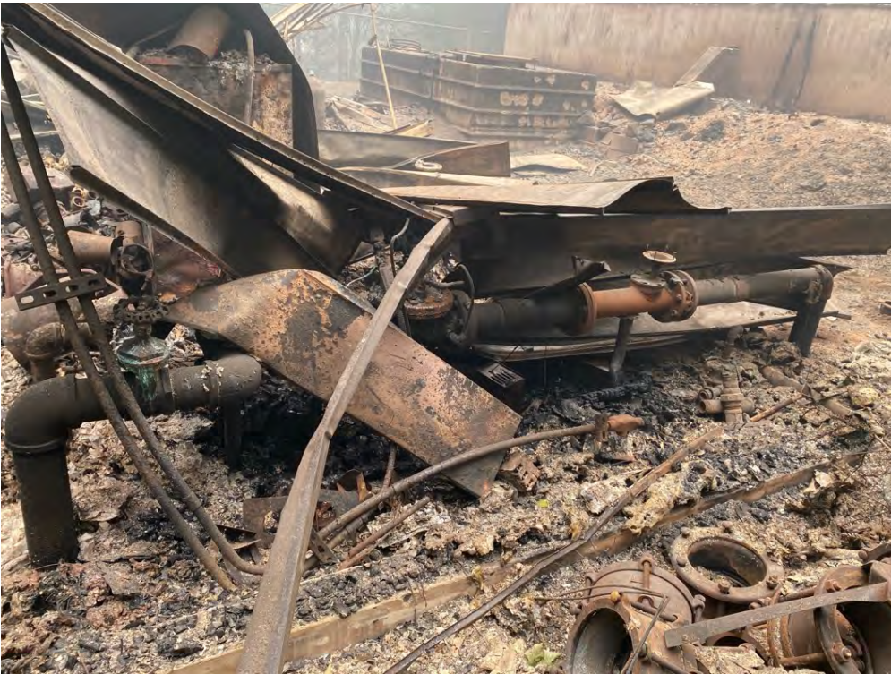
Figure 6: Damage to a pump station at the City of Detroit, OR (Photo credit: Heath Cokeley, Oregon Association of Water Utilities Circuit Rider).
